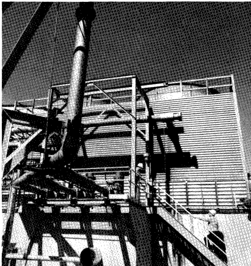
FIG. 1. Biological cooling tower shown under construction at Lever's Edgewater, N.J., plant. Piping in left foreground supplies water from cooling tower to edible process department.
